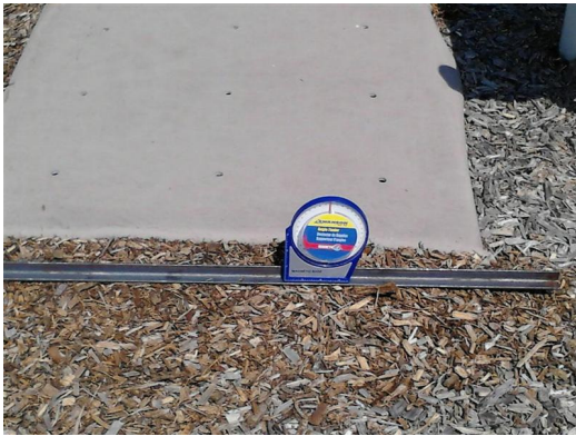
(Picture after backfilling around mat)
